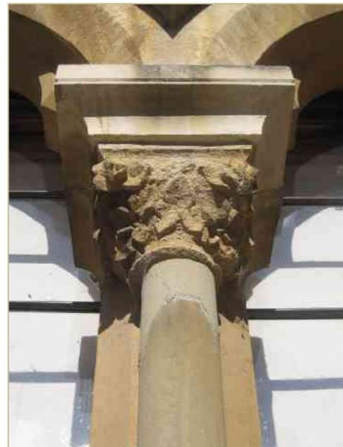
**Figure 13. Damage to capital on southern tower of western elevation**
