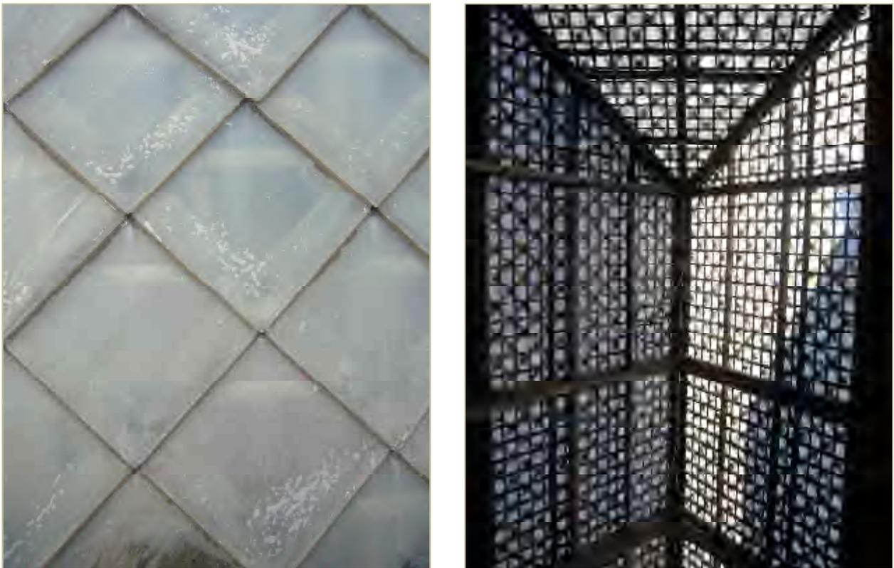
**Figure 19. Left, detail of the glass slates from above. Right, the effect of the glazed roof from below**
