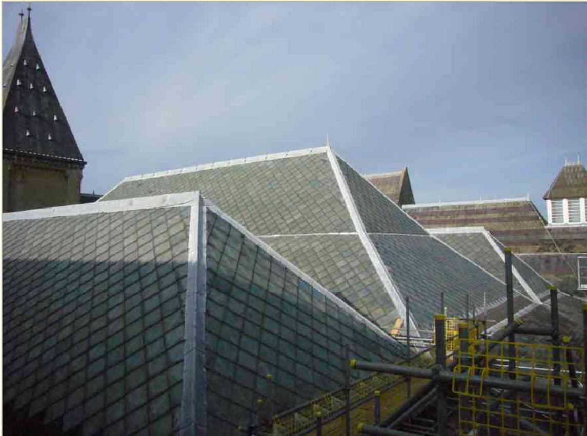
**Figure 14. The glazed roof from above facing north-westwards. Also note the banding of the slates on the roof to the rear right of the image**
