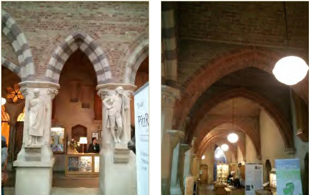
**Figure 20. Left, brickwork and banded stone arches on the western end of the central court. Right, barrel vaulting along the ambulatory at the western end of the central court**
