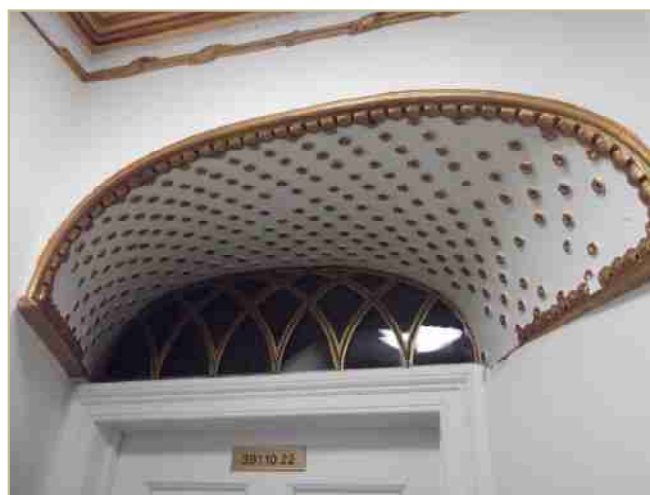
Figure 17. Historic details picked out in modern decorative scheme
