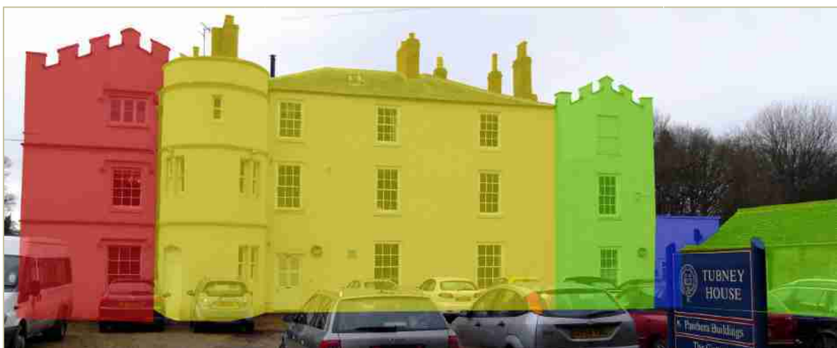
Figure 9. 9.1, top, modern ground floor plan. 9.2, middle, southern elevation looking northwards. 9.3, middle, northern elevation looking southwards. Throughout the c.1521 Gollds is highlighted in red, the 1811 extension is highlighted in orange, the c.1840 extension is highlighted in yellow, the c.1861 extensions are highlighted in green, early 20 th -century extensions are highlighted in light blue, and 21 st -century extensions are highlighted in dark blue
