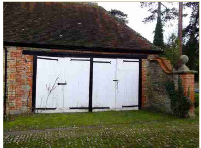
Figure 15. 15.1, left, the South Lodge looking from the southeast. 15.2, top right, the southern elevation of Cottage One is on the right of the image, the eastern elevation of the Panthera buildings is at the left of the image. 15.3, bottom right, garage doors and ball finial gateposts at eastern end of Cottage One
