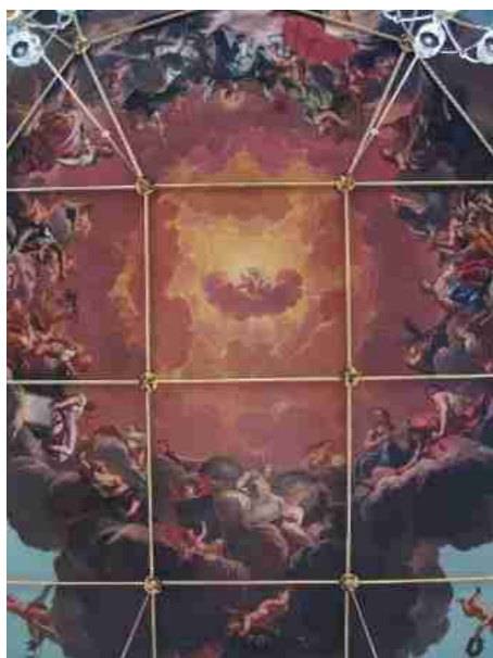
Figure 5. The restored ceiling
