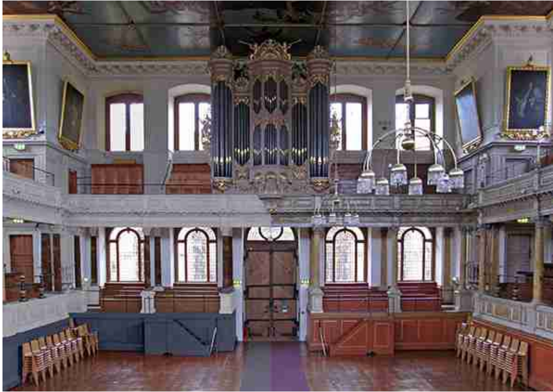
Figure 4. The interior of the Sheldonian, showing Wren’s original colour scheme (restored in 2011) on the left and the nineteenth-century colour scheme and intrusive twentieth-century light fittings on the right. Note the heavy marbling on the balconies on the right-hand side, and how on the left-hand side the darker pillars blend in with the background.
