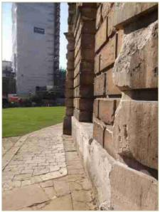
Figure 27 Left, weathering to rusticated stone base, note repaired cornice. Top right, repairs to stonework on ground floor. Bottom right, damage to stonework on ground floor
