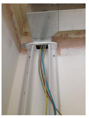
Trunking Connecting trunkings using bushes is not acceptable.
