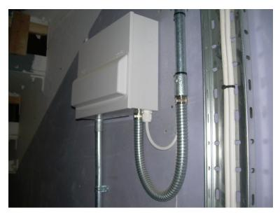
Kopex should be used in an appropriate manner i.e. for connections between isolators/plug and sockets and vibrating equip
