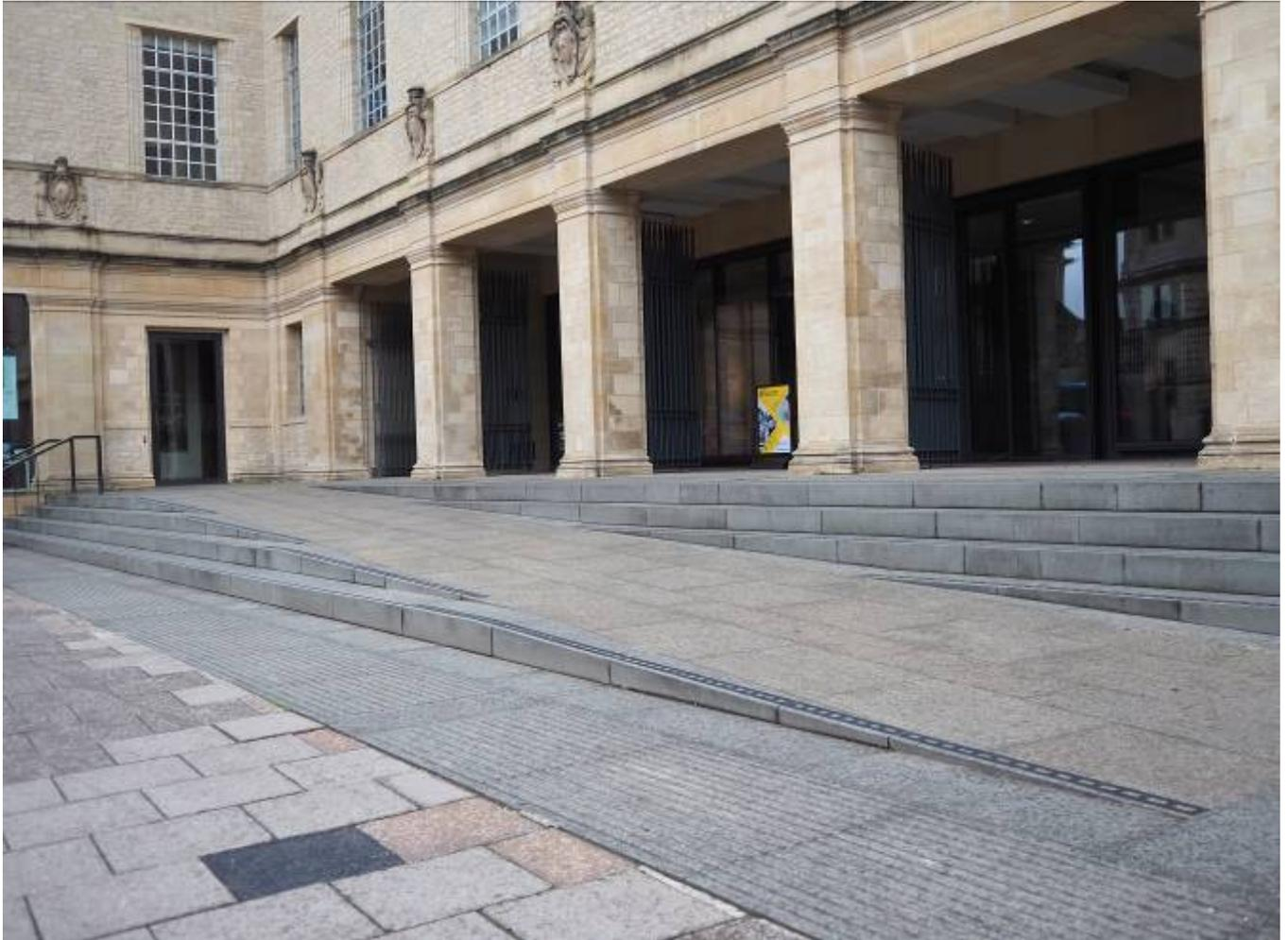
Ramps which cut through steps must be carefully designed to minimise the risk of trips
